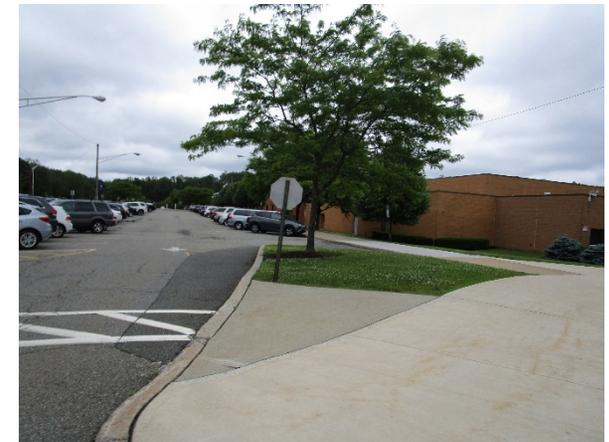
Parking spaces in the parking lot to the southeast of the building can be converted to pervious pavement to capture and infiltrate stormwater runoff from the parking lot. Additional parking spaces throughout the site could be retrofitted as well. A small bioretention system can be installed adjacent to the shed to manage the rooftop runoff. A preliminary soil assessment suggests that the soils have suitable drainage characteristics for green infrastructure.
