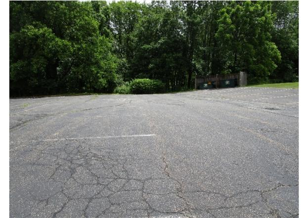
Pervious pavement can be installed in the northeast portion of the parking lot to capture and infiltrate stormwater runoff from the parking area. A preliminary soil assessment suggests that the soils have suitable drainage characteristics for green infrastructure.
